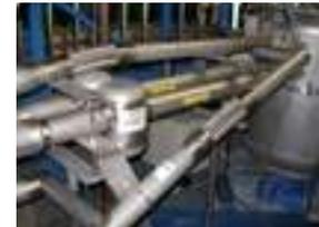
CERN-LHC: Local cryogenic distribution system for liquid Nitrogen and liquid Argon supply to calorimeters of ATLAS instrument (transfer lines + valves boxes).
